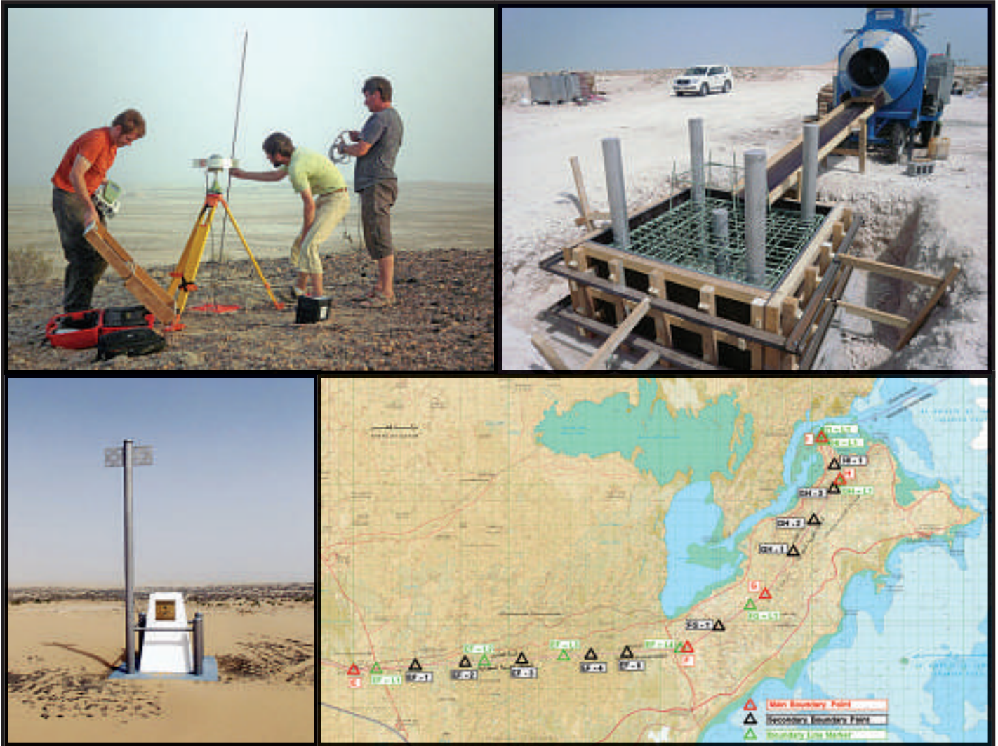
Border work for Saudi Arabia/Qatar – clockwise from top left: Geodetic control survey for the demarcation of borders (IGN FI: 1996/2000 and 2007-2010 © D Bordon/IGN); construction of a boundary marker (IGN FI: 1996/2000 and 2007-2010 © J-C Poyard/IGN); position of the new border markers on the border map (IGN FI: 2010-2011); and intermediary boundary marker (IGN FI: 1996/2000 and 2007-2010 © C Romieu/IGNFI)
